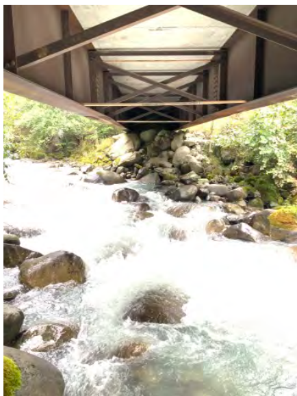
Left Bank Abutment when facing downstream
