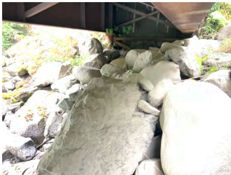
Right Bank Abutment when facing downstream
